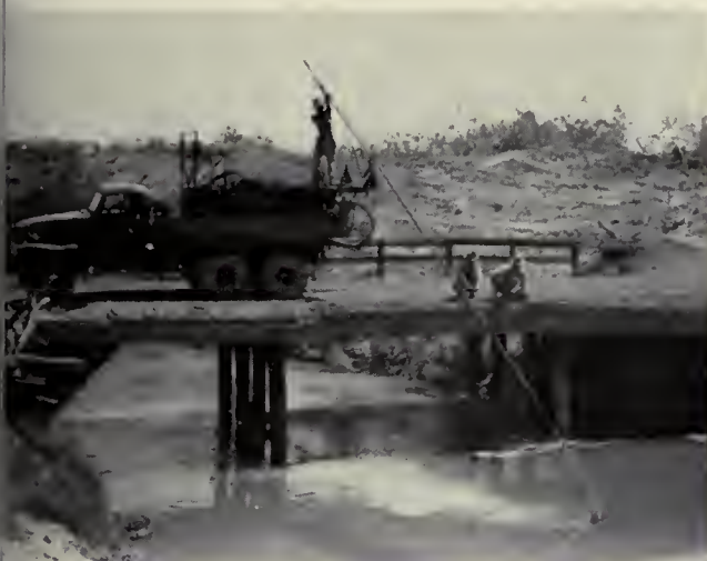
INHIBITING ALGAE IN ARIZONA (at left) by large-sized spray loaded with Rada. Below, masses of moss (see arrows) at Yuma's Boundary Pumping Plant being pulled up by weed hooks, before Rada made the job easier. Photos by the author.
